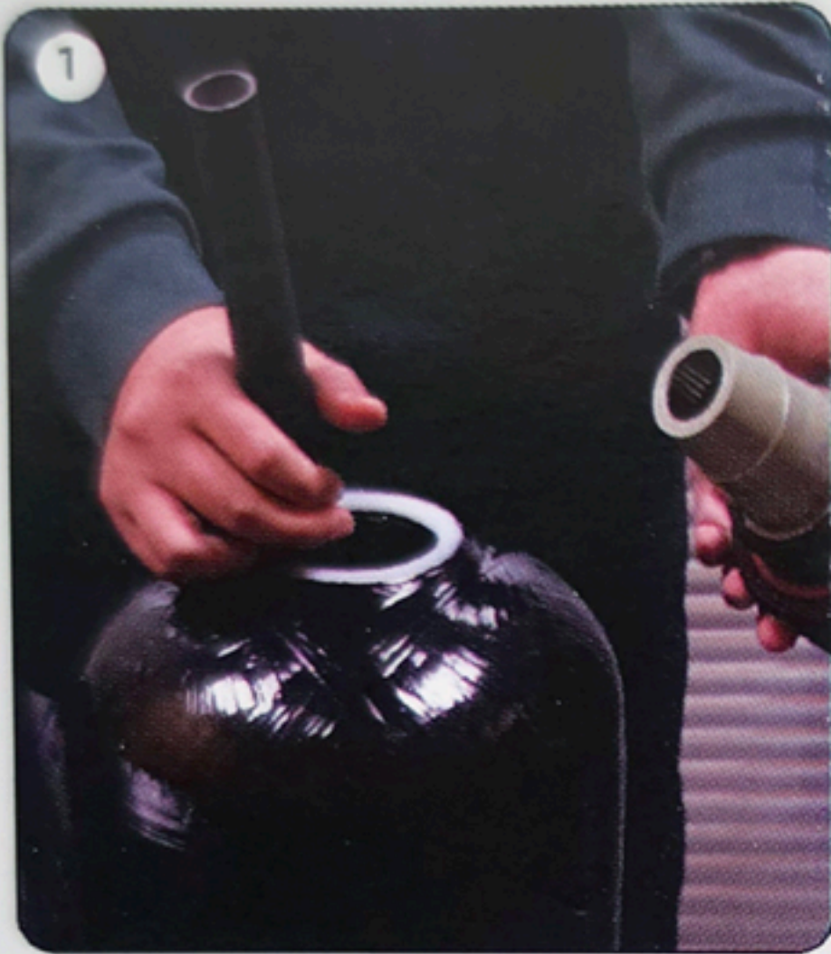
Pulling out the riser tube
